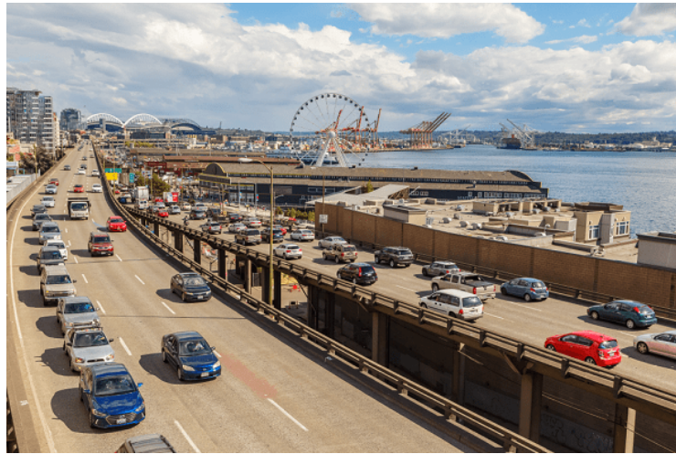
Figure 6. View from Above of Alaskan Way Viaduct
