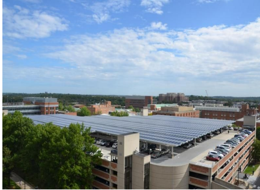
Figure 7: Solar Parking Canopy at University of Maryland
