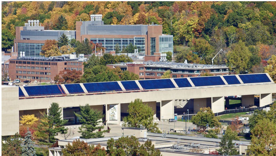
Figure 6: Solar Parking Canopy at University of Massachusetts Amherst
