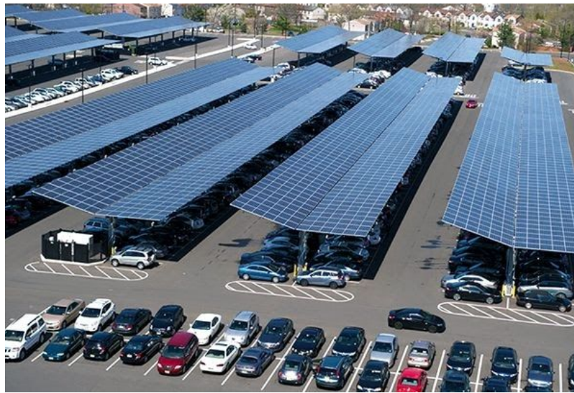
Figure 15: Rows of Raised Rectangular Strips of Solar Panels
